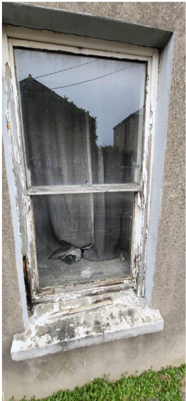
Images I & J from 12 th February 2025. Vegetation growing along the façade, paint work peeling from door and window, and window showing signs of rotting. No change in the condition of the property at 2 Manor Hill.
