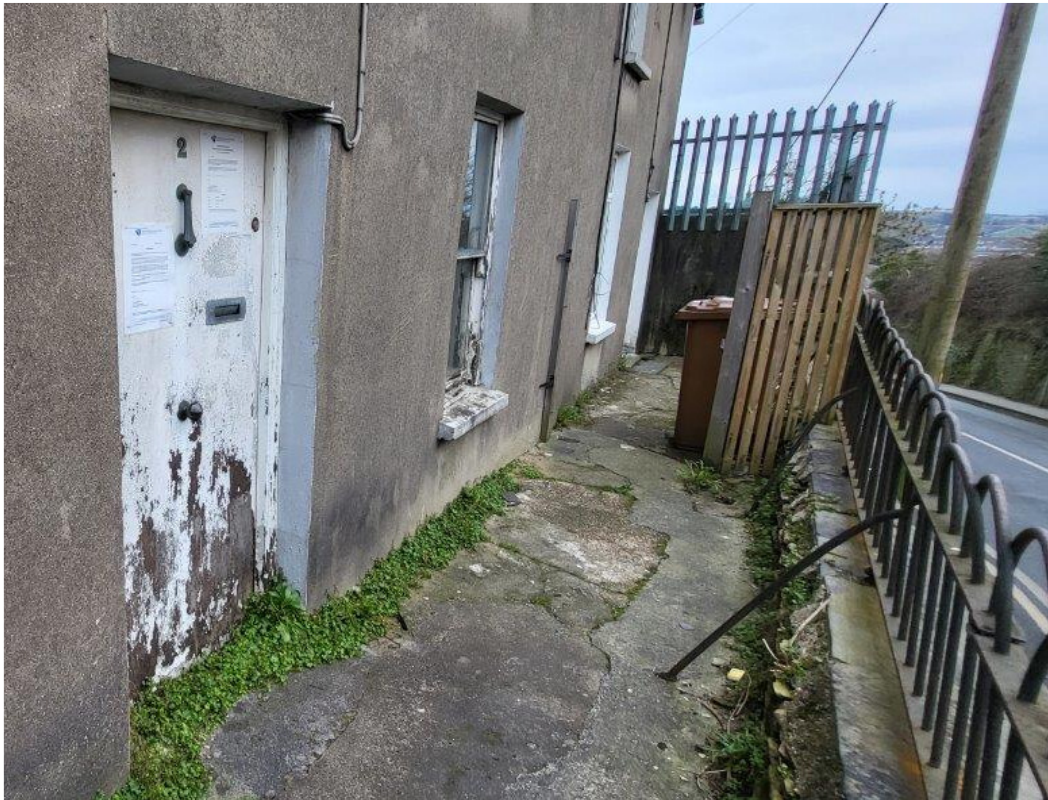
Images I & J from 12 th February 2025. Vegetation growing along the façade, paint work peeling from door and window, and window showing signs of rotting. No change in the condition of the property at 2 Manor Hill.
